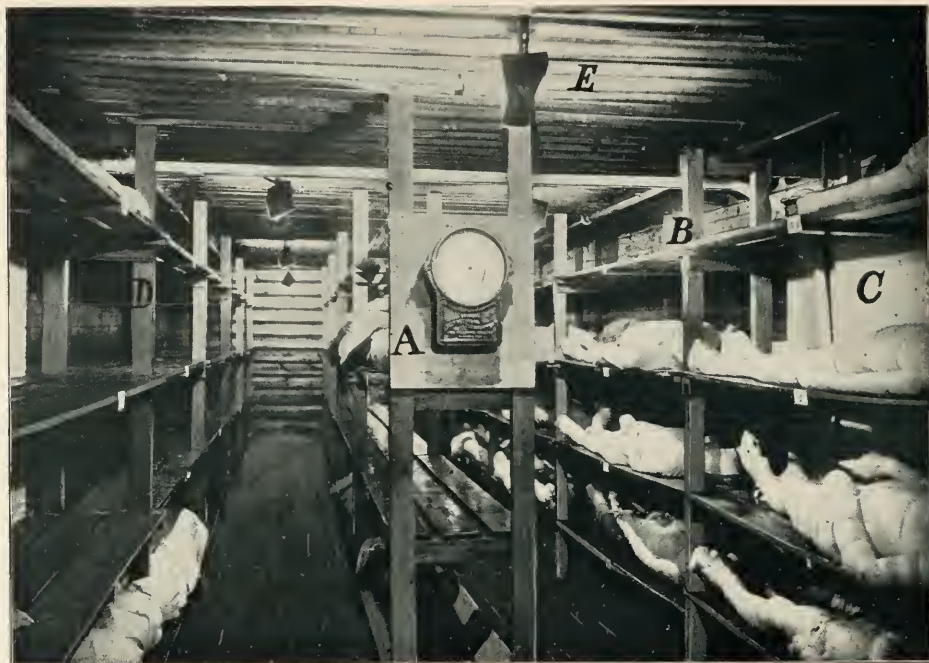
FIG. 181.—Refrigerating room. A , recording thermometer and middle tier of shelving; B and D , tiers of shelving; C , brine tank; E , pipes of refrigeration apparatus.
